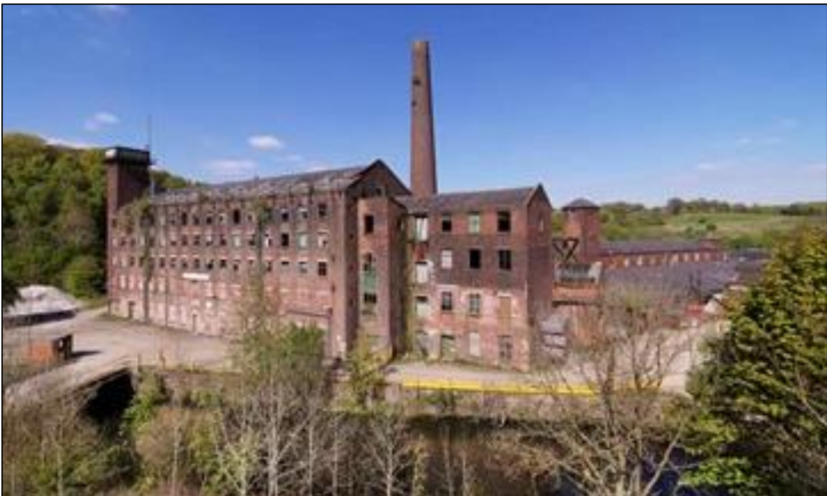
Plate 10 Looking east towards Crimble Mill from within the Site
