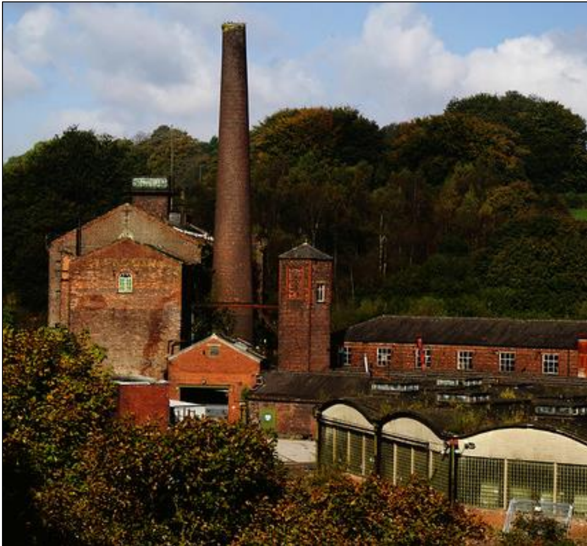
Plate 11 Looking north towards Crimble Mill from Crimble Lane
