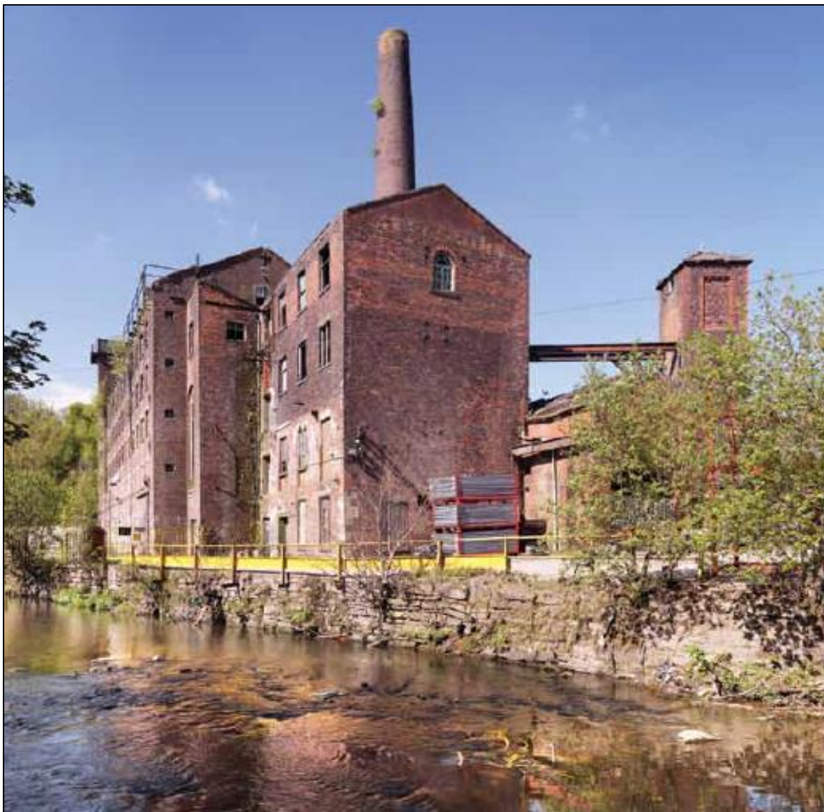
Plate 8 Looking north towards Crimble Mill from the River Roch
